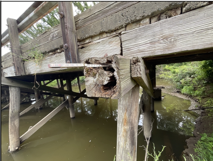
Bent 8 above pile 4 the timber cap has decayed and is hollow 5' deep
