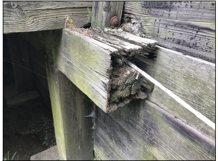
Bent 1: left end of cap hollow up to 2'-6"
