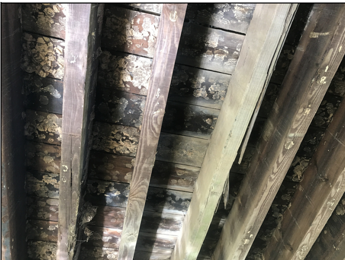
Span 4 girders 8&10 have splits and checks
