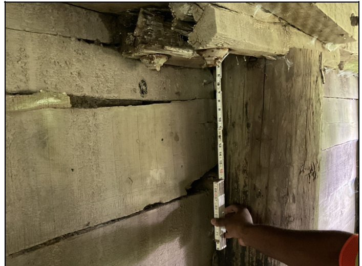
Bent 17 the splice on the cap above pile 3 is crushing and hollow allowing the cap to sag 1 1/2"
