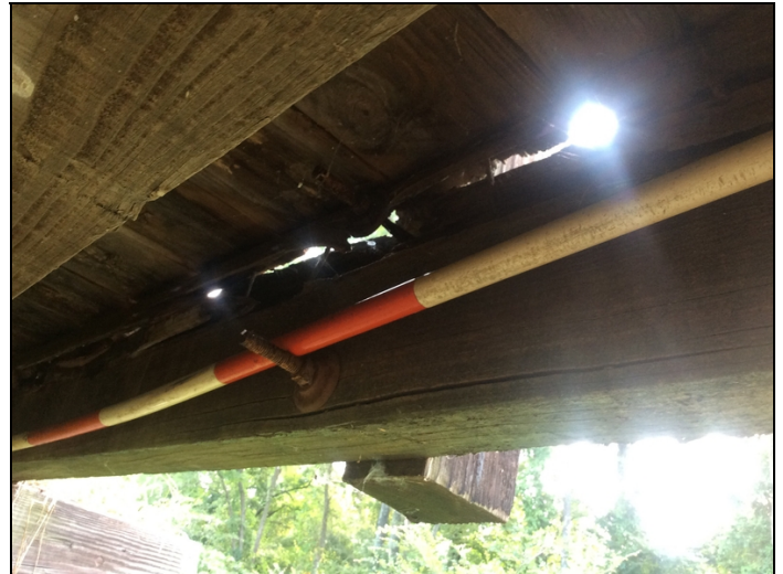
Span 16 girder 1 hollow and crushing the entire length.
