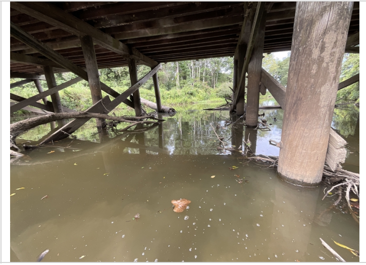
Logs and drift bents 3,4,5
