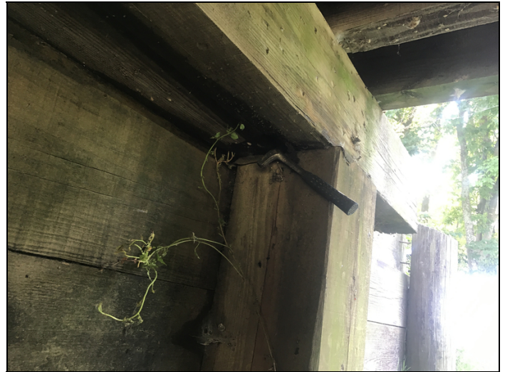
7 foot of the left end of bent 1 cap is split and hollow over pile 1.
