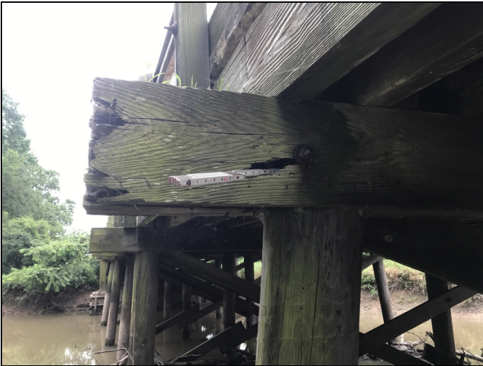
Bent 3 left end of cap is hollow past pile 1.
