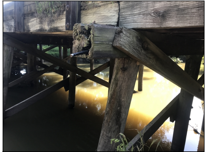
bent 8 right end of cap is decayed and hollow the 3 1/2' over pile 4
