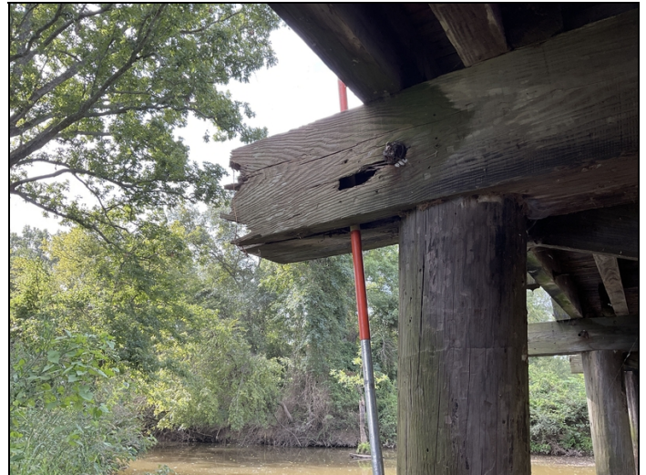
Bent 3 cap decayed and split at left end
