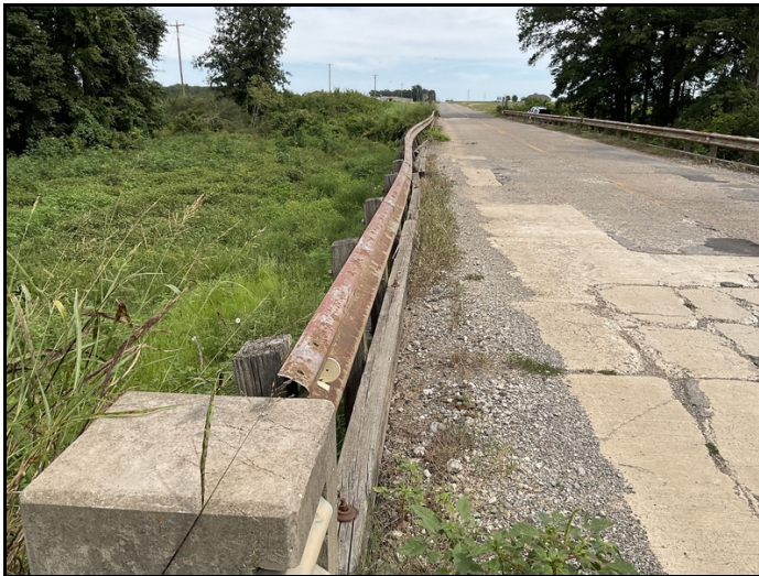
Guardrail damage on west side
