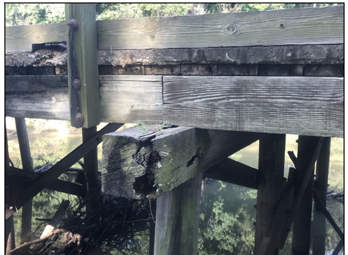
Bent 3, left end is decayed and hollow past pile 1.
