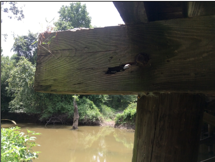
Bent 3, left end of the cap, decayed and hollow.
