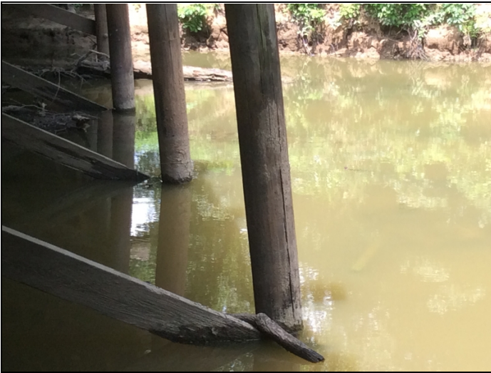
Bent 7, pile 1, large cracks.
