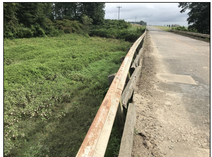
60' of bridge rail is damaged from traffic impact on right side of bridge
