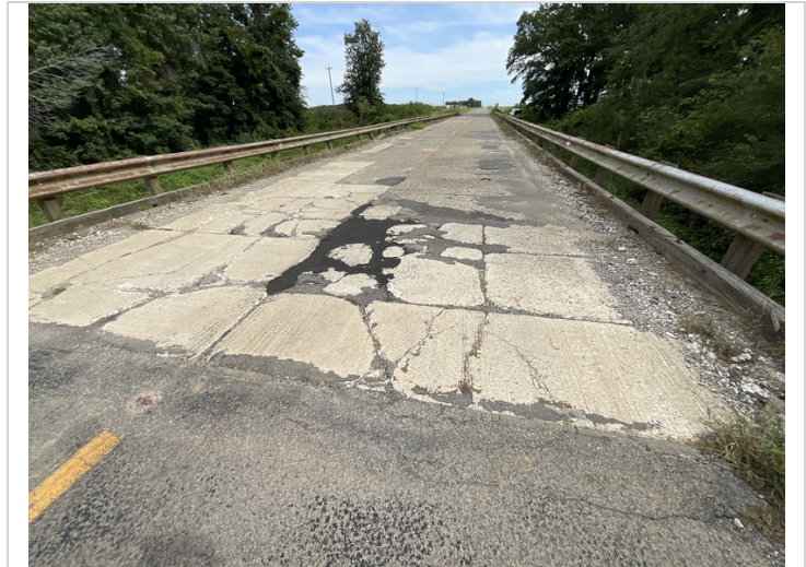
Concrete patches filled with asphalt
