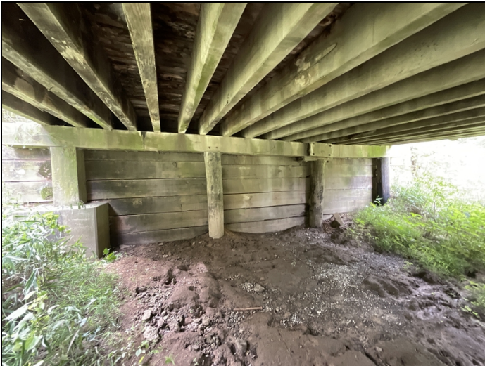
Bent 17 abutment the timber cap has settled 1 1/2 due to decay at the cap splice over pile 3
