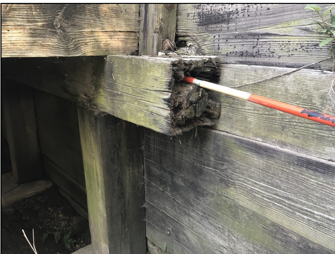
Bent 1: left end of cap hollow up to 2'
