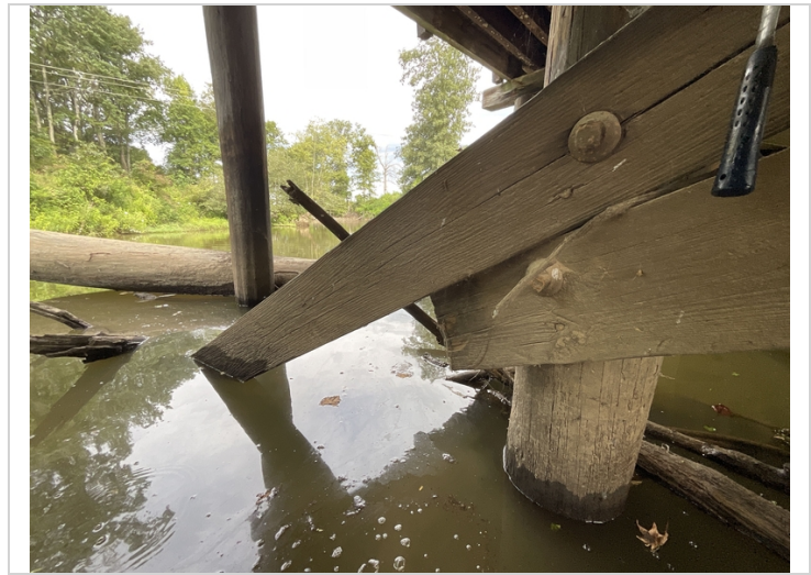
X brace at bent 5 has broken loose from pile 4 at bottom
