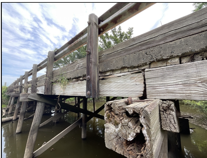
Span 7 outside girder 18 is decayed and split
