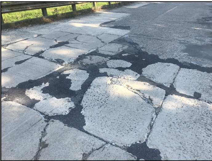
Span 16 spalls and spall filled with asphalt
