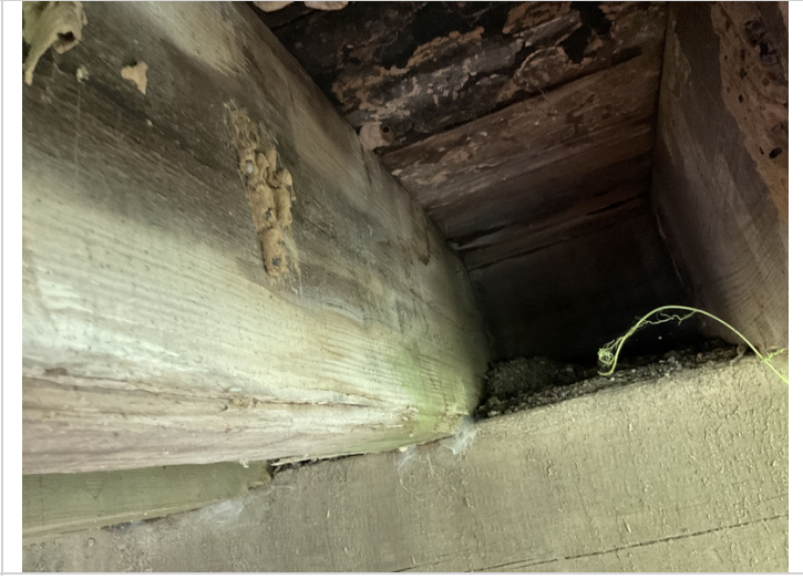
Bent 1 timber girders decayed at ends
