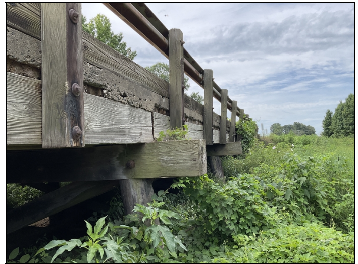
Outside girders on west side are no longer supporting the guardrail post allowing free movement
