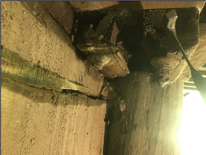
bent 17 the cap splice connection is decayed and crushing over pile 3
