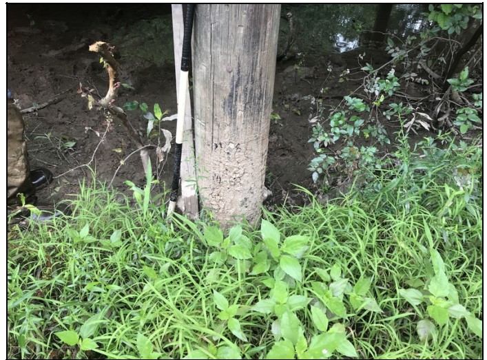
Bent 14 pile 4 is decayed on bottom 2'
