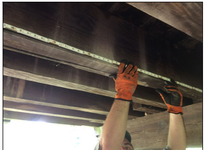
Spain 2, girder 15, cracked.
