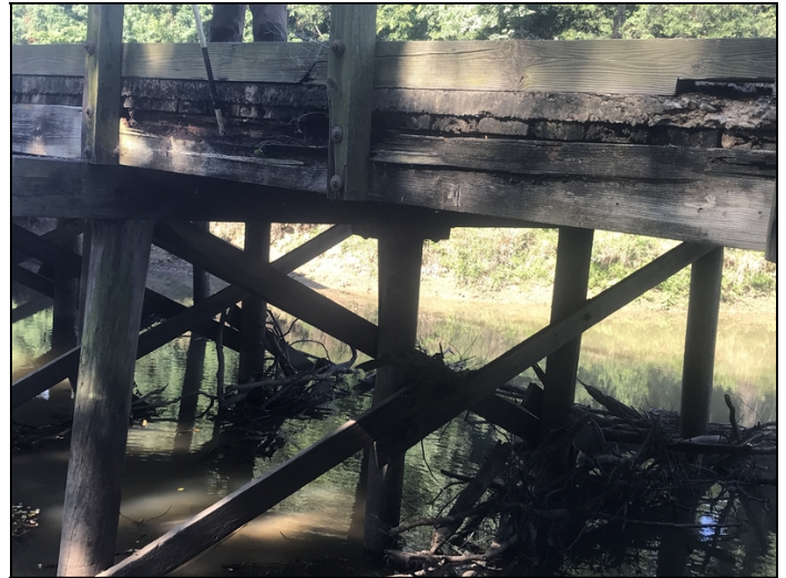
span 3 girder 1 is rotted the whole length
