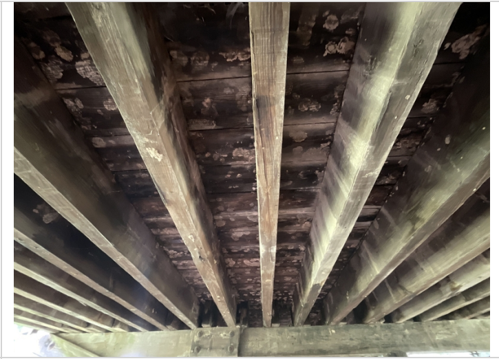
Span 15 girder 10 has split mid span
