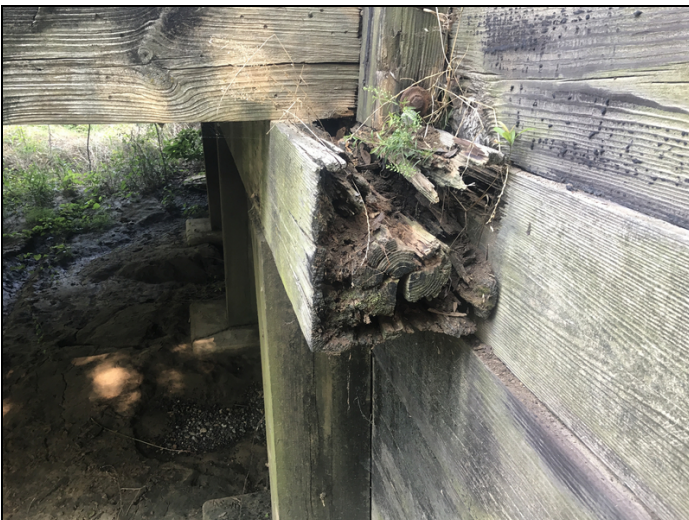
Bent 1 left end of cap is split and hollow over pile 1
