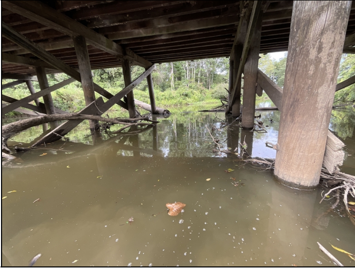
Logs and drift bents 3,4,5
