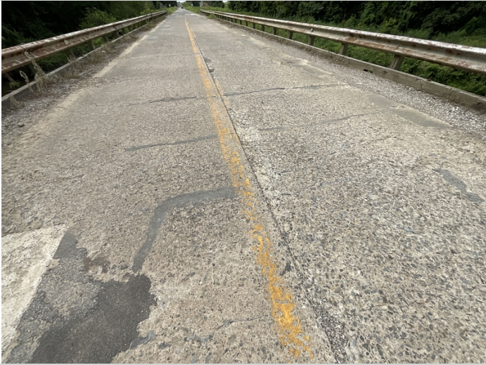
Spalls and abrasion in the deck in multiple locations some cracks have been sealed
