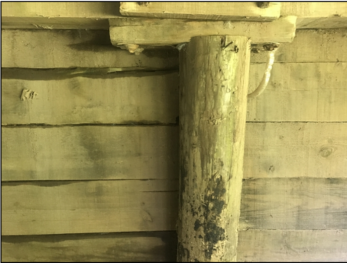
Bent 17 pile 3 is hollow at the top
