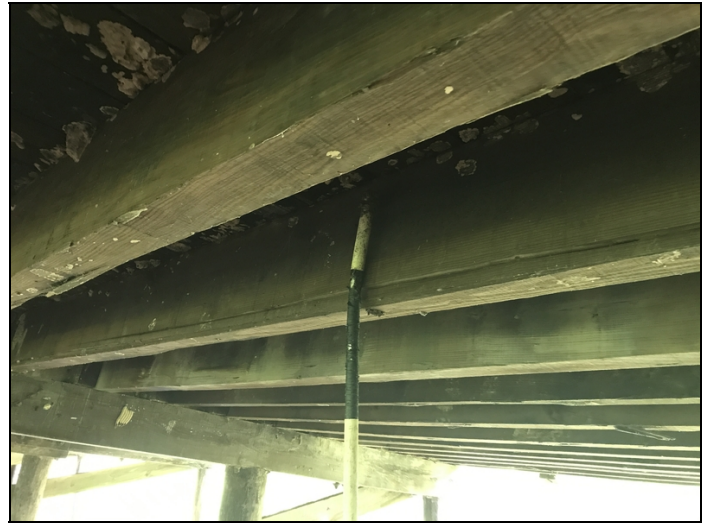
Span 13 girder 9 is cracked along 10' of bottom.
