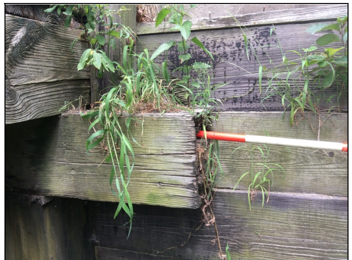
Bent 1, left end of cap, decayed and hollow 1 1/2 feet.
