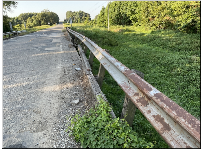
Right side bridge rail damage
