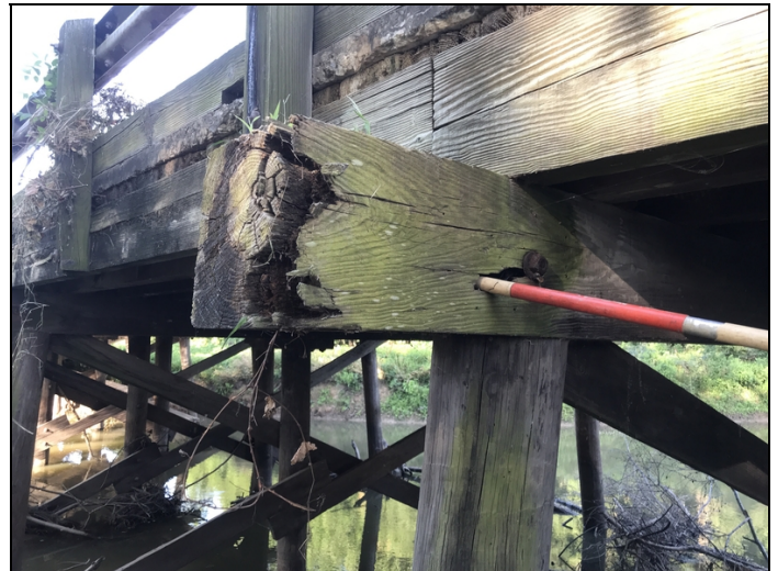
Bent 3: left end of cap hollow. It's hollow 3' from the end of the cap past pile 1.
