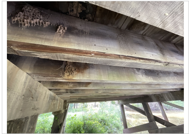
Span 2 girder 15 split at bent 2
