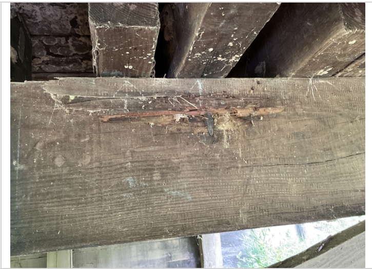
Bent 2 cap under girder 5 has a split where spike has been nailed
