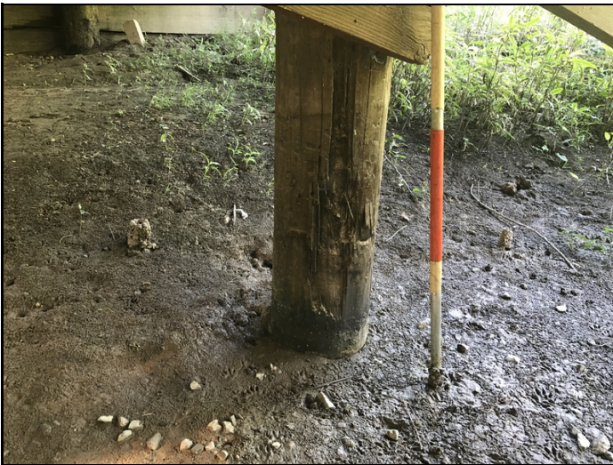
Bent 16, pile 3 with a large shake
