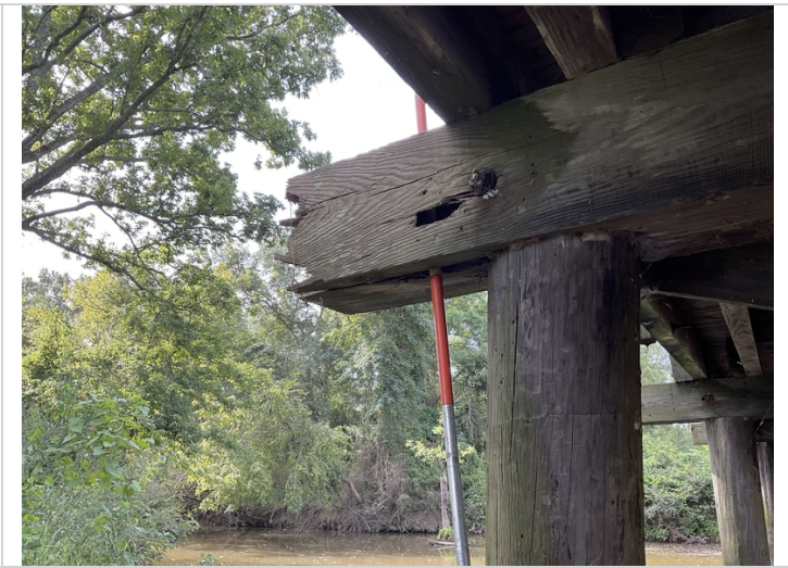
Bent 3 cap decayed and split at left end
